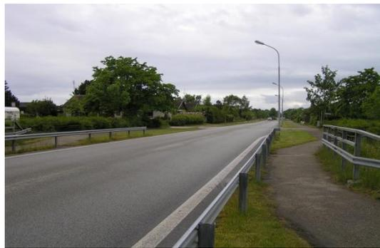
Figure 5 "SCAFT-separation" on a street with high speeds and low use of separations
